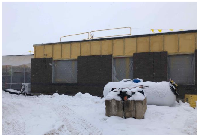
Installing masonry at Admin Addition
