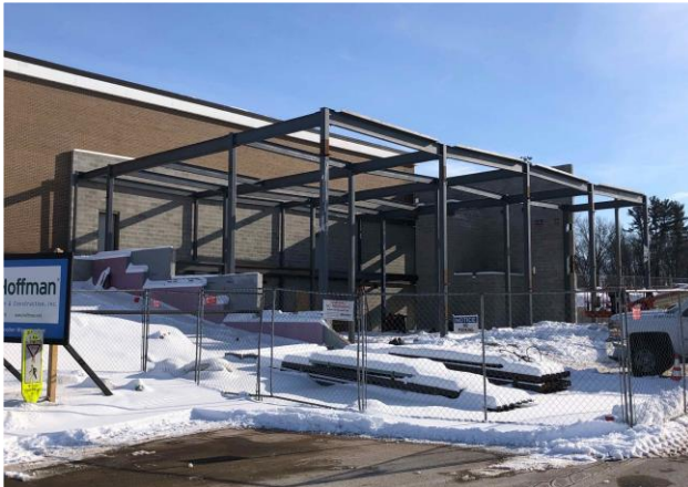
Set structural steel at Fitness Addition
